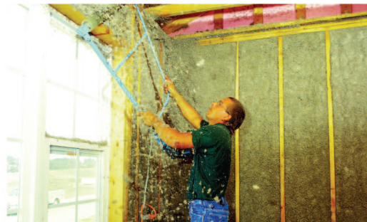
An installer “shaves” excess wet-spray cellulose fiber insulation from wall studs after it has dried.
